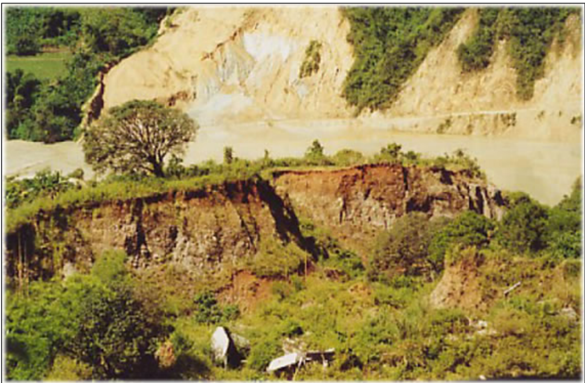
Photo: Save the Abra River Movement Massive ground subsidence from mining in Colalo, Mankayan. The white structures at the bottom are remains of the Colalo Elementary School, 1999.
